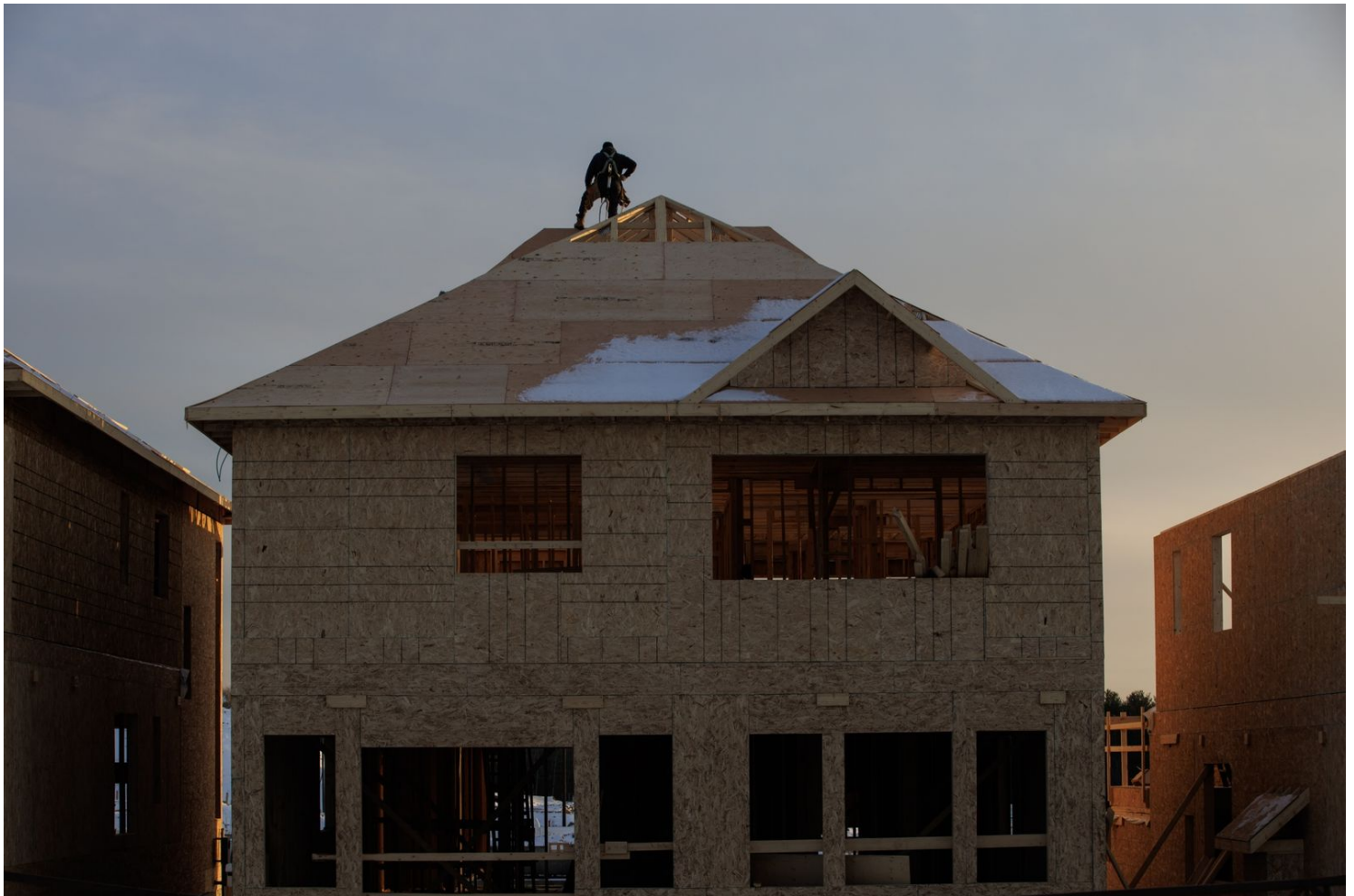
A home under construction in Vaughan, Canada. Photographer: Cole Burston/Bloomberg
