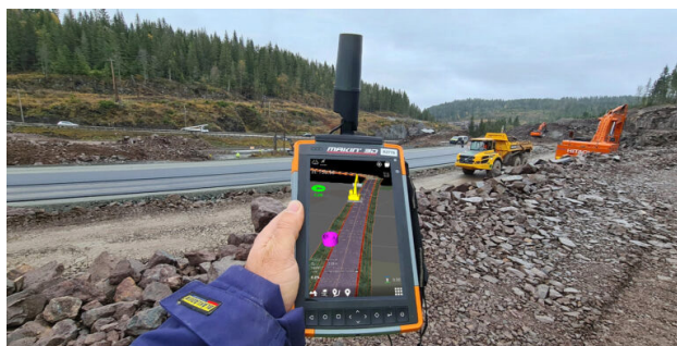
A surveyor uses a Makin GNSS-enabled tablet to verify road alignment and grade as crews place aggregate along a highway construction corridor. Image courtesy of Elationtech.
